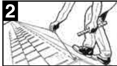
Snap chalk line on rear side of the ridge (or whatever side of the ridge that aesthetic considerations dictate) and no more than one inch (1") from the peak. **Note:** Important to clear center ridgepole before cutting. See diagram below.
