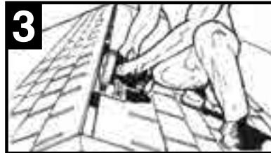
Cut along chalk line. Remove roof sheathing. **Note:** Slot should not be cut any closer than within twelve (12) inches of gable end, hip intersecting ridge.
