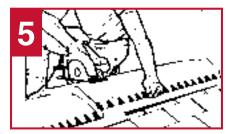
Nail each additional section in the same manner until entire ridge is covered. A chalk line may be utilized to ensure vent alignment. Cut last piece to length and install with original uncut end to the outside.
