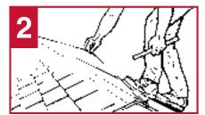
Snap chalk line on both sides of the ridge and no more than .750 (3/4) of an inch from the peak. **Note:** If a ridgepole is present, cut a wider gap to allow a minimum of 1/2" air gap on both sides of the pole into the attic space - but do not remove more than 2-1/4" of roof sheathing material from either side of the ridge.
